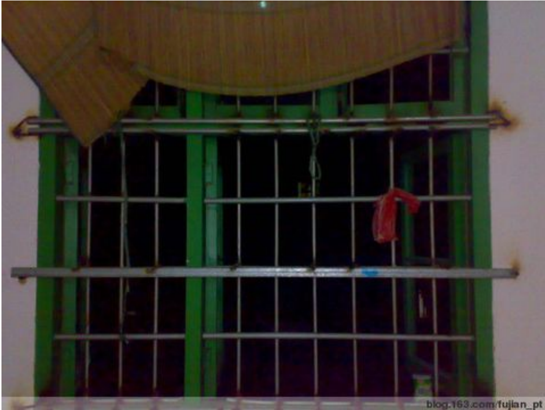
Bars of the cells for detention in the Family Planning office of Yuanzhuang Town, Xianyou County.
